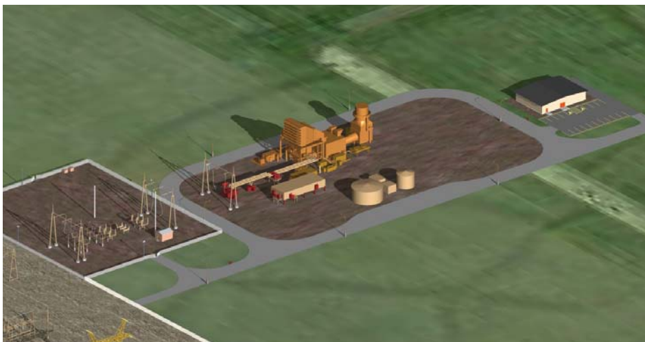
This rendering of the Charles D. Lamb Energy Center that will be built in Kay County, Oklahoma shows the 103-megawatt simple-cycle combustion turbine-generator in the center, the administration building on the right and the substation on the left.
